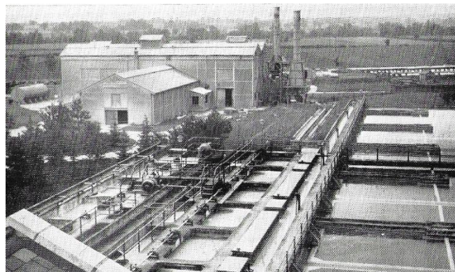
Foreground – the Mixing Tanks and Sedimentation Tanks. Background – The Lime Recovery Plant.
