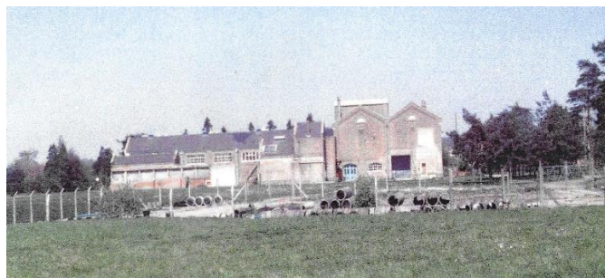
The Old Treatment Works before demolition
