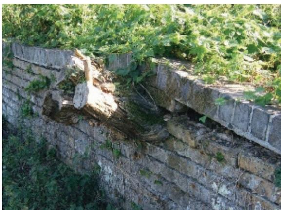
The platform had fallen into a pitiable state of neglect, with roots growing through the engineering bricks, and the platform crumbling under the invasion of ivy and other creepers.
